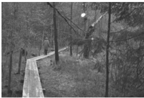
On-going trail and bridge work. Details next Bog Notes!
